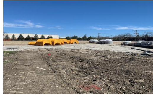
Truck Parking lot Expansion
